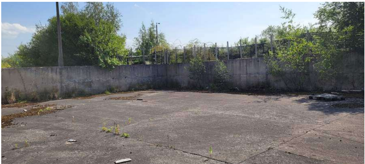
Reinforced Concrete Wall
