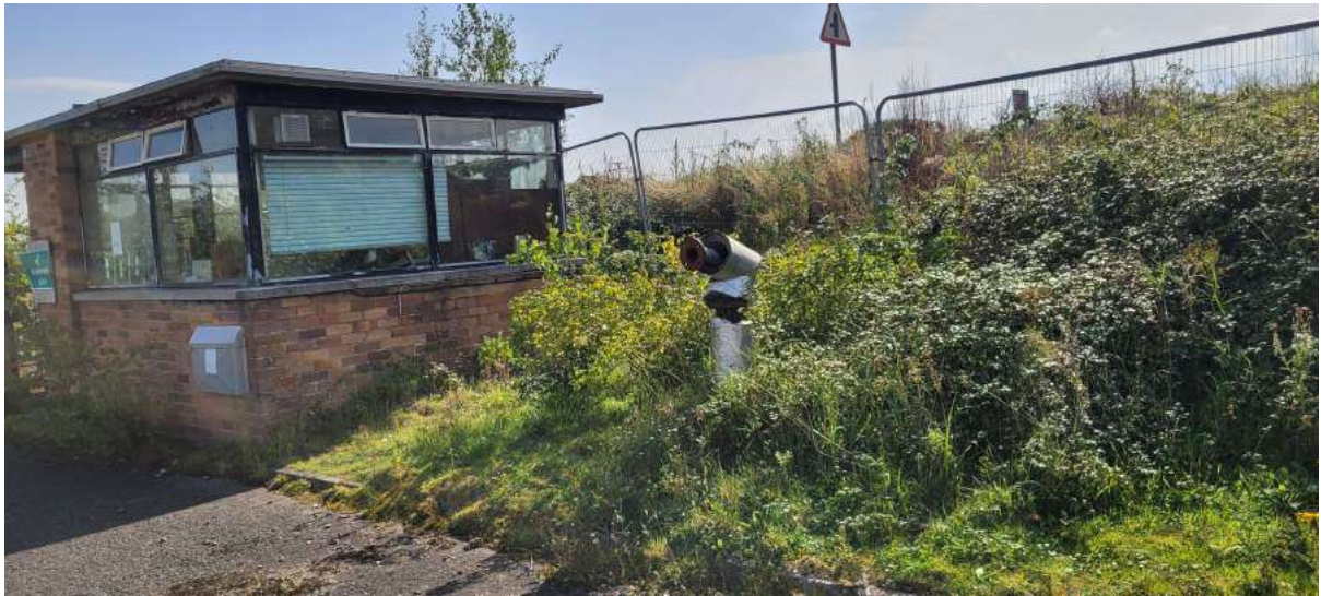
Former Gate House – Note Steam Pipe
