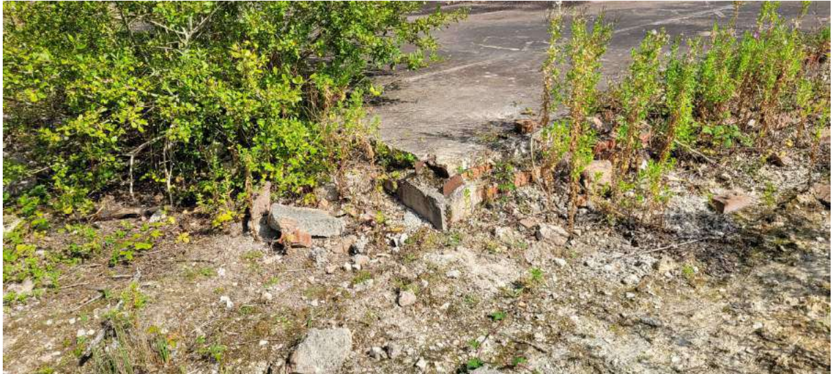
Former Building Positions – Existing Slabs Remain
