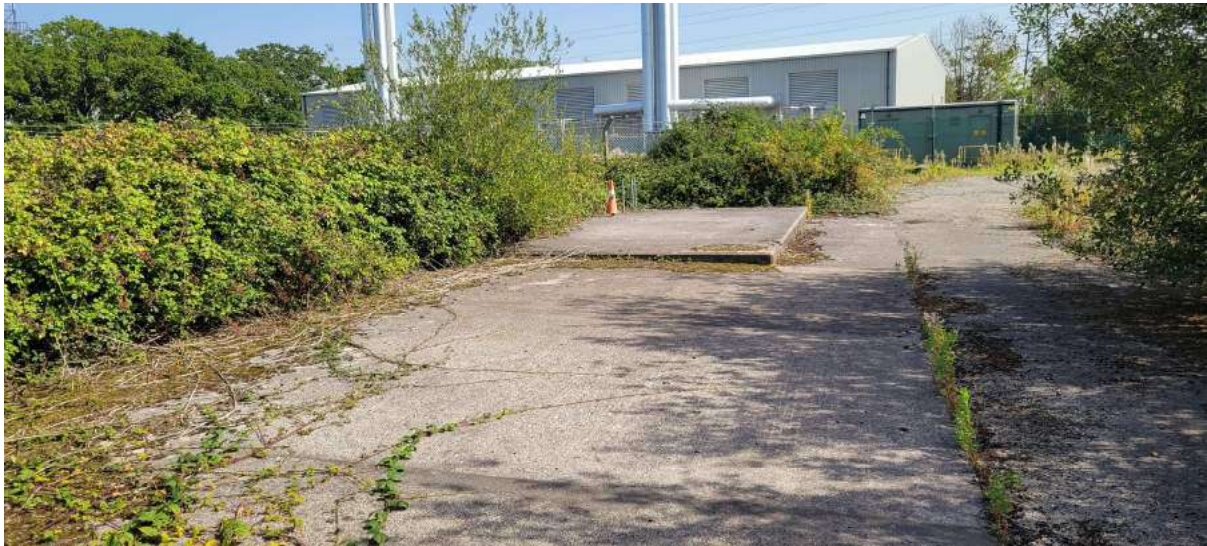
Concrete Roadway and Raised Platform (Note Gas Power Station in Background)
