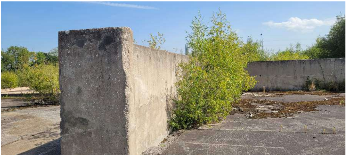
Reinforced Concrete Wall
