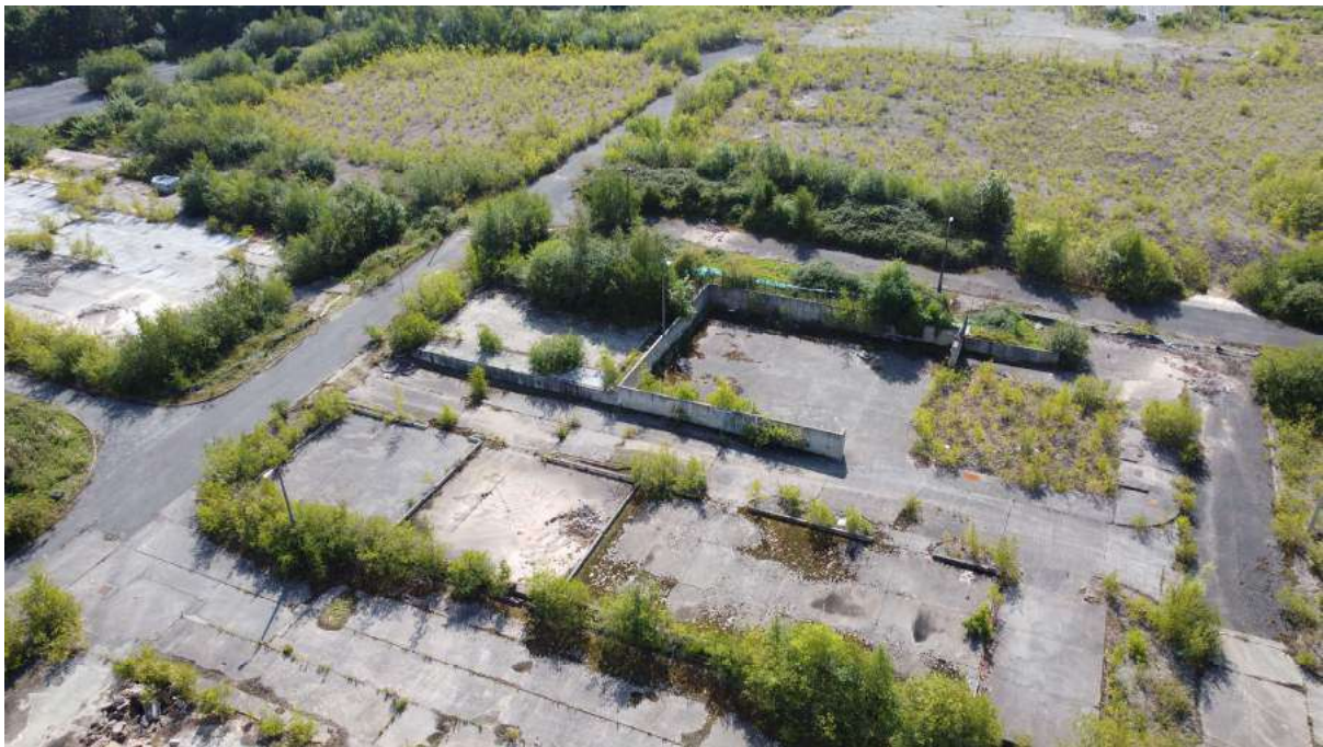
Concrete Walls, Platforms and Retaining Structures
