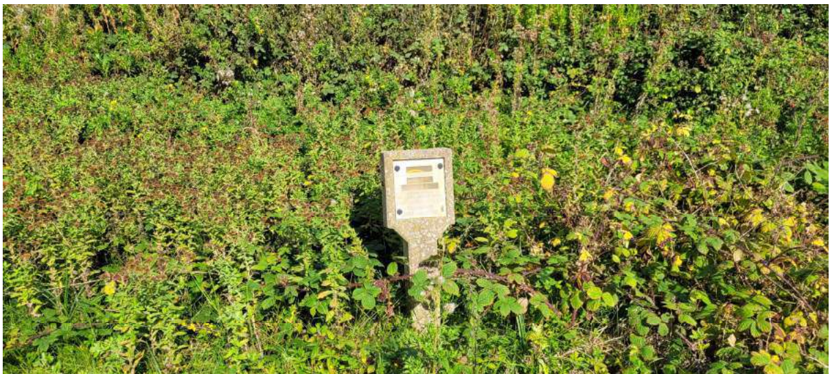
Gas Main Marker
