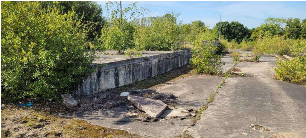
Concrete Platform – Suspected Former Loading Bay
