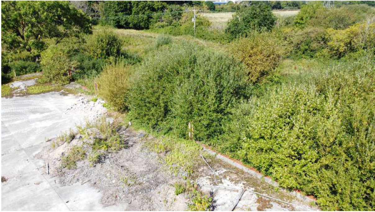
Partially obscured retaining wall & Steel Stanchions.
