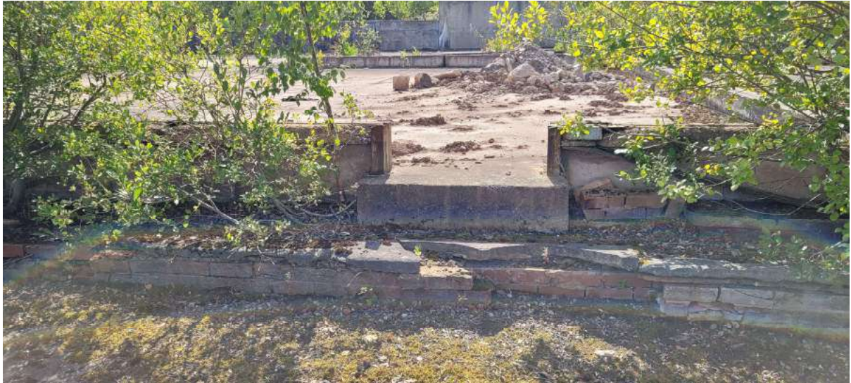
Former Threshold and Level Changes
